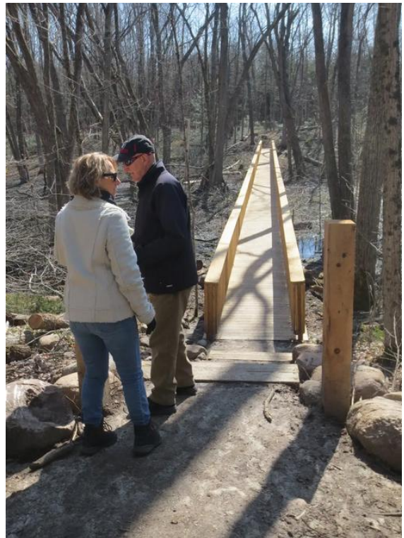
THE NEWLY COMPLETED HI-LO BRIDGE IS A BEAUTIFUL STRUCTURE WHICH SHOULD LAST A LONG TIME. QUINTE CONSERVATION DID A GREAT JOB IN BOTH THE FUNDRAISING AND THE CONSTRUCTION. PHOTO AND CAPTION BY TED PORDHAM.
