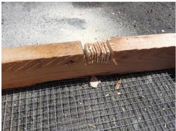
2. Using an electric skill saw set at a depth of 2.5 cm, make many cuts within the 5cm section.
